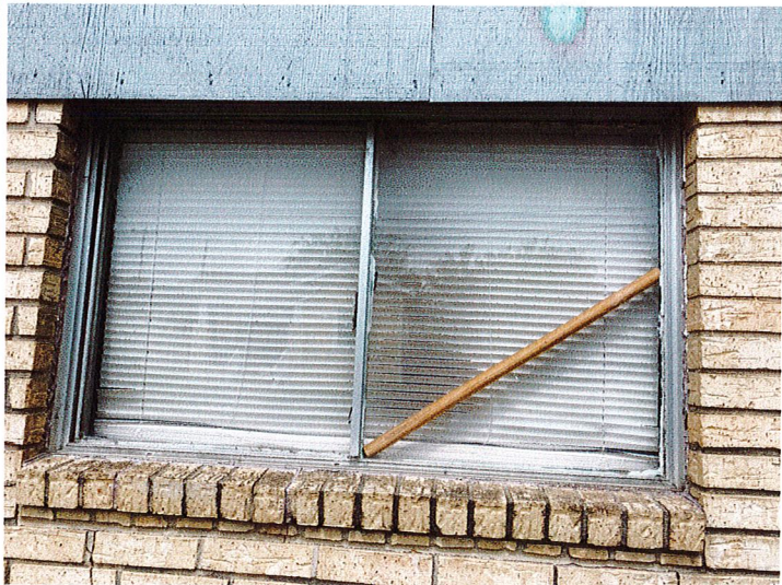
Flooring destroyed during foundation work, windows inoperable, glass broken
