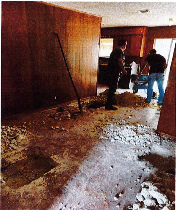
Flooring destroyed during foundation work, windows inoperable, glass broken
